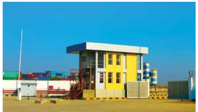
Smart Gate Complex
