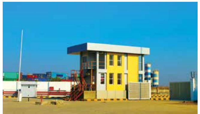
Smart Gate Complex
